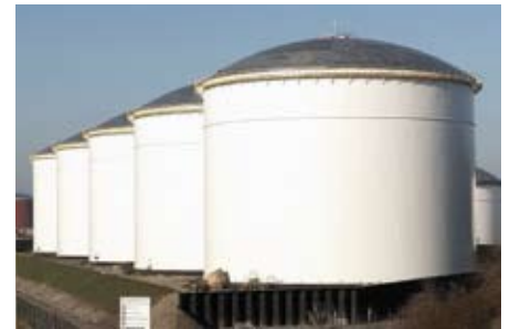
Five new jet fuel tanks
