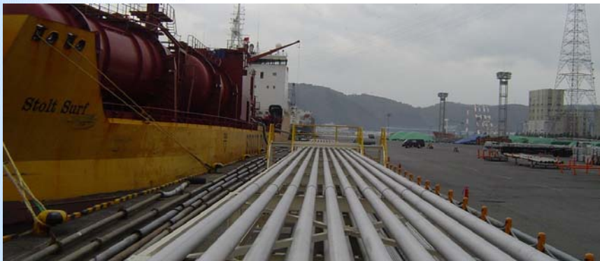
New permanent jettylines at pier 6 in Ulsan
