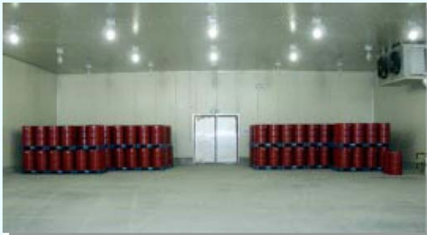
Cooling of drummed MDI in Vopak's first "frozen" warehouse
