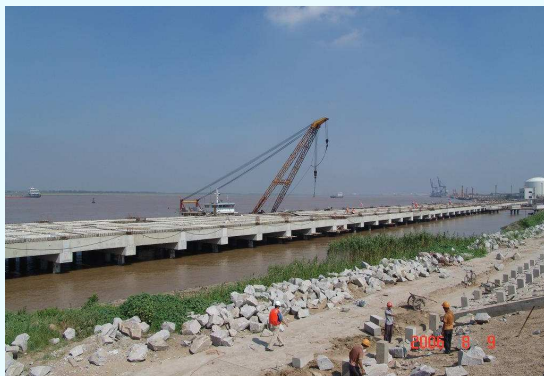
Civil work for the jetty is on schedule
