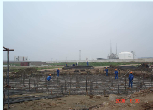
Preparation of the tank foundation
